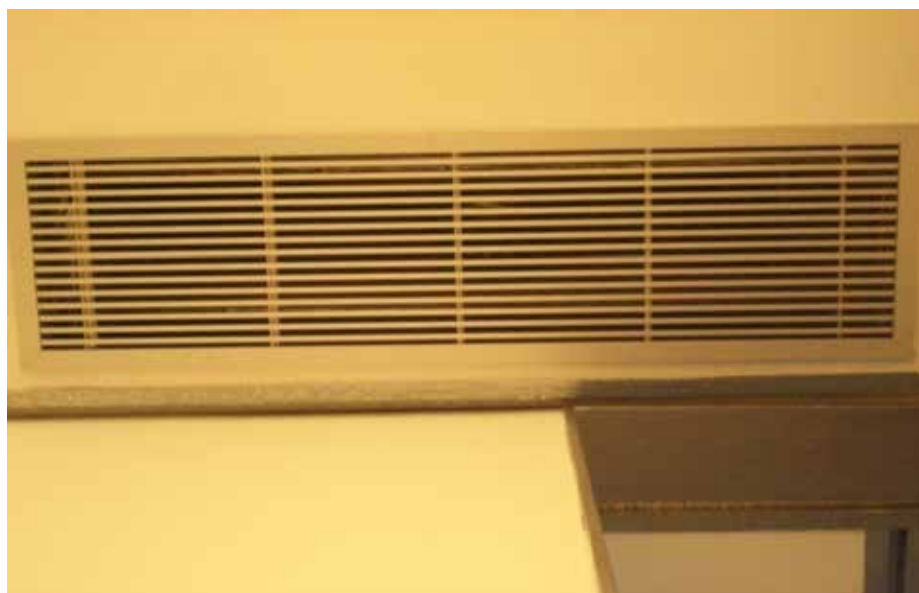
Horizontal clima on the top of the wall
