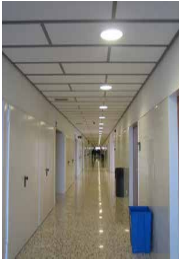
Fluorescent lamps along the corridor
