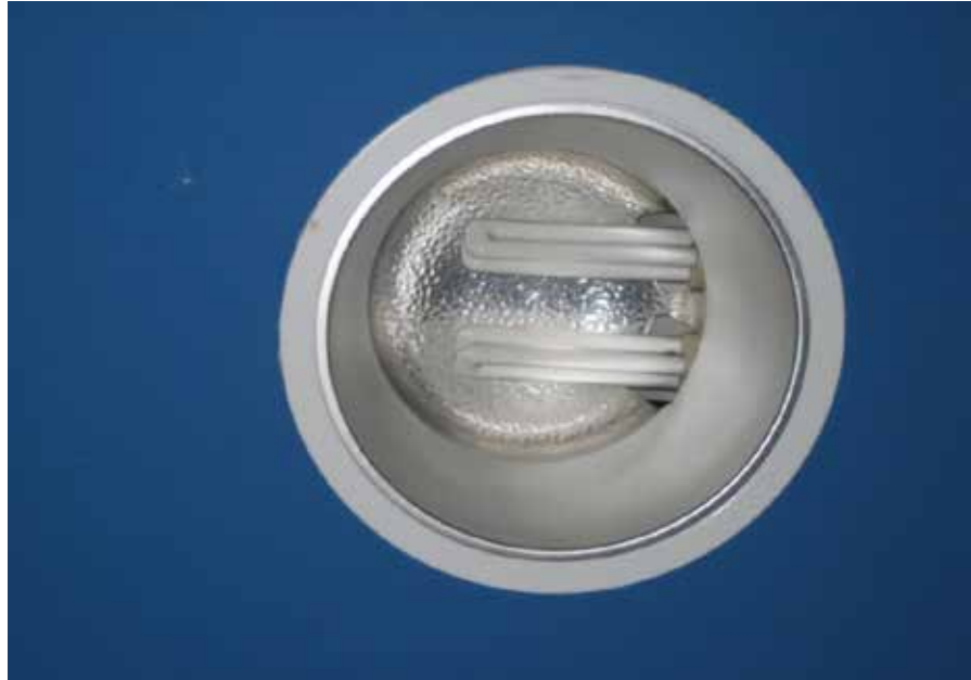
Fluorescent lamp d=0.20\text{m} , 16watt/lamp ( 2*16=32\text{watt} )
